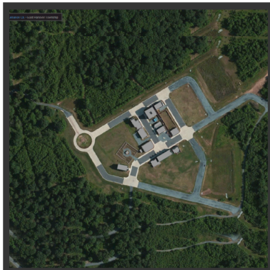
Figure 1. Aerial view of the FTIF test facility.
