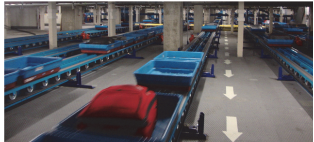
Figure 1: A conveyor is used to store baggage trays while providing random access. This scenario can be vastly improved with the system shown in fig. 2
